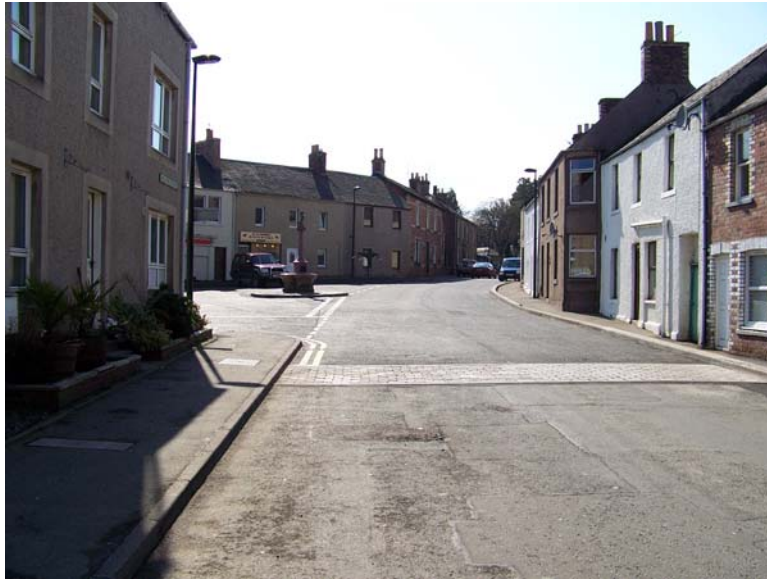
Path & Road surfacing Improvements and new lighting to Cross area
