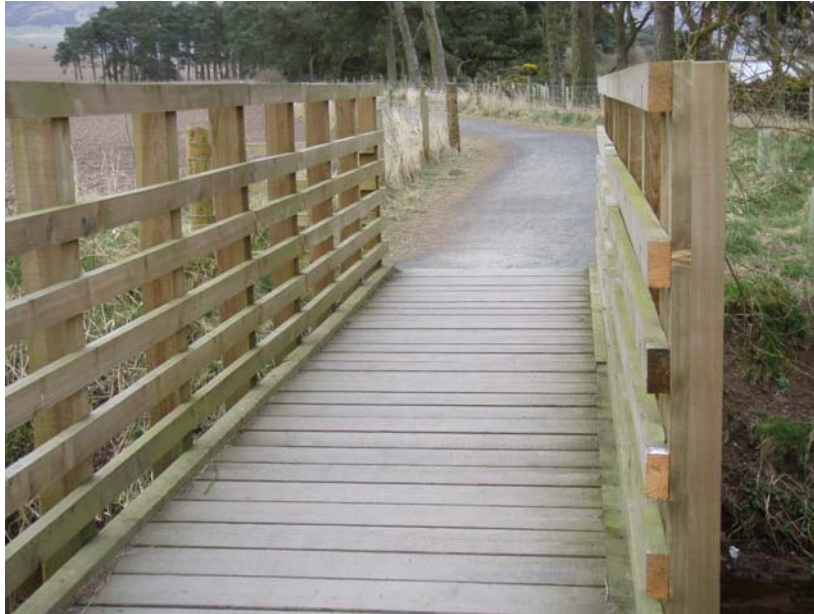
A bridge installed on the Loch Leven Heritage Trail
