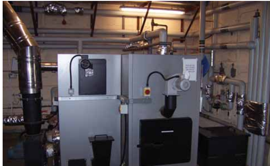
Figure 1.1 Biomass boiler
