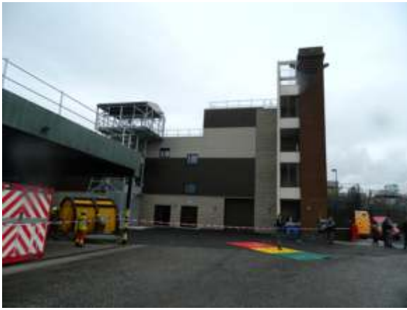
The new training facilities at Kingsway East Fire Station provide the backdrop for fire crews to participate in an exercise involving a chemical spillage, search and rescue of casualties and decontamination.
