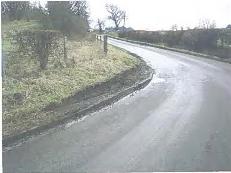
Photo 1 – Verge Damage at Bend at Tullibardine
