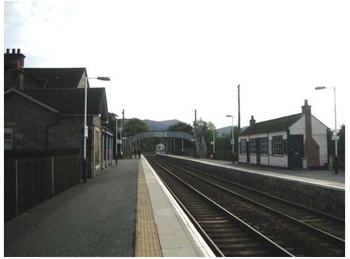
Railway Station & Footbridge
