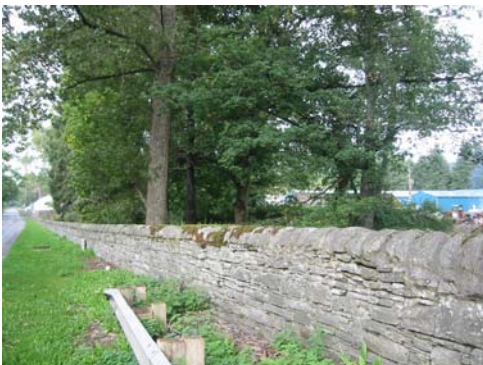
Distinctive use of rubble and dressed stone, slate and timber.
