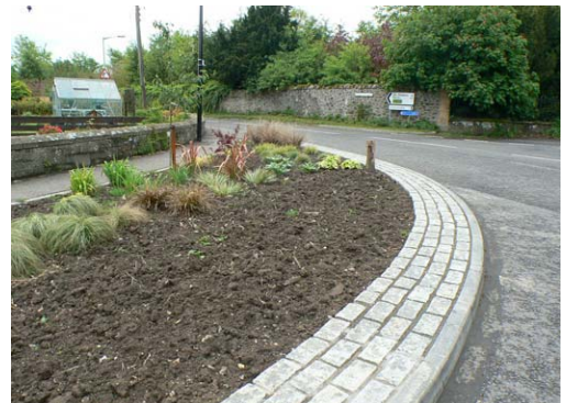
Newly planted border edged in traditional setts, St. Madoes Road, High Street junction
