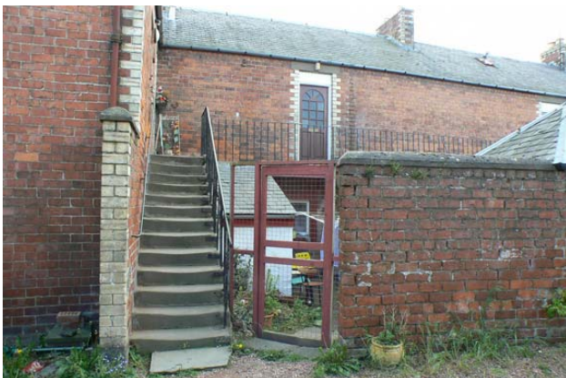
External stair with platt access to upper tenements, Cowgate Southbank
