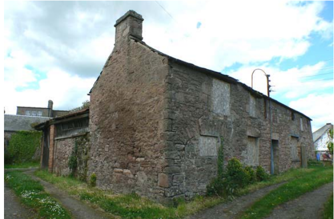
Ancillary building located to the rear of Dalgleish House
