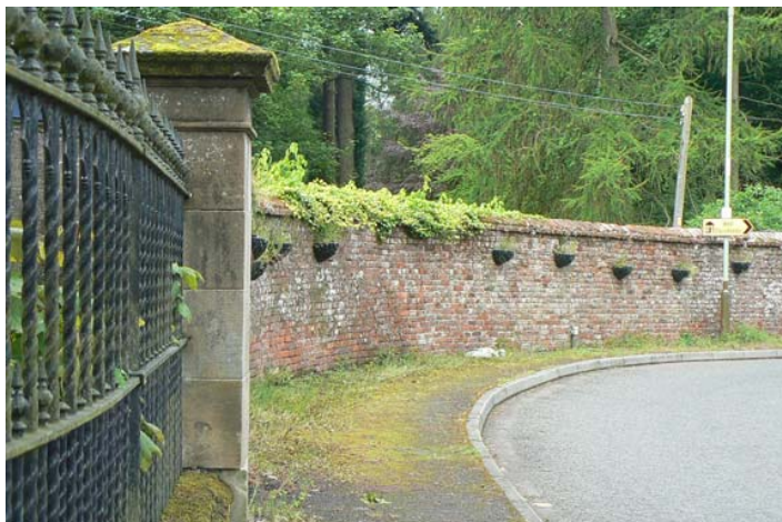
Curving brick boundary wall of Errol Park with decorative ironwork and stone piers
