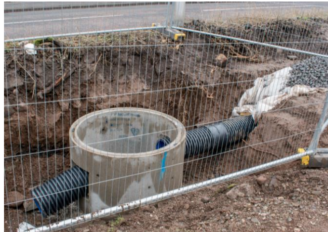
Cricket Pitch – Construction of drainage system
