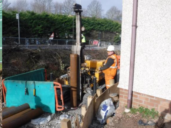
Lochty Park – installation of tubular piles (that will form the foundation of the flood wall)
