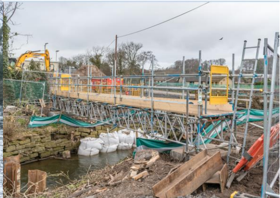
Low's Works Cottages/Brockhill – Installation of temporary service diversion bridge
