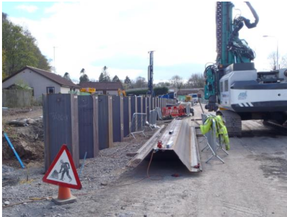
Lochty Park - installation of sheet pile flood wall
