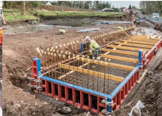
Trout Farm – Erection of reinforcement and shuttering for flood wall bases
