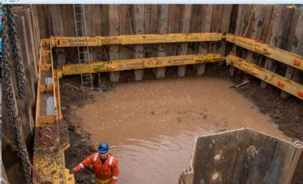
Vector – Installation of temporary sheet piles to construct pumping station chamber
