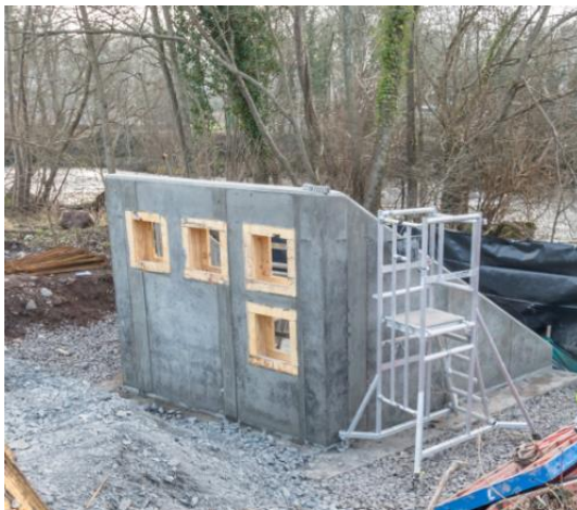
Trout Farm – Pumping Station outfall (the gaps are for pipes)
