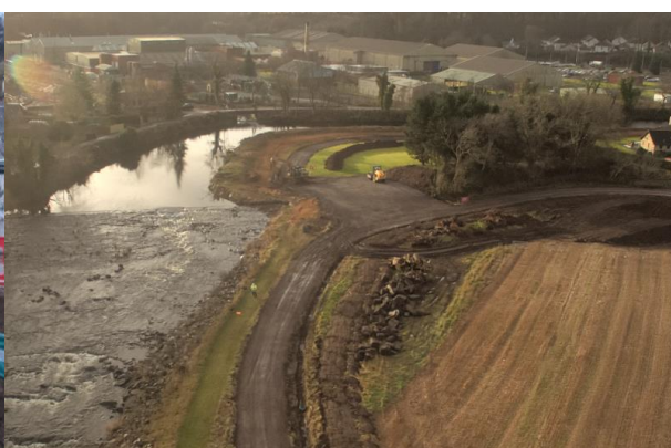
Deer Park/Craigneuk - Construction of haul/access roads adjacent to Low's Weir for construction of flood embankments
