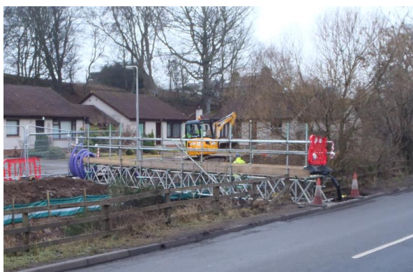
Lochty Park - Installation of temporary utility diversion bridge
