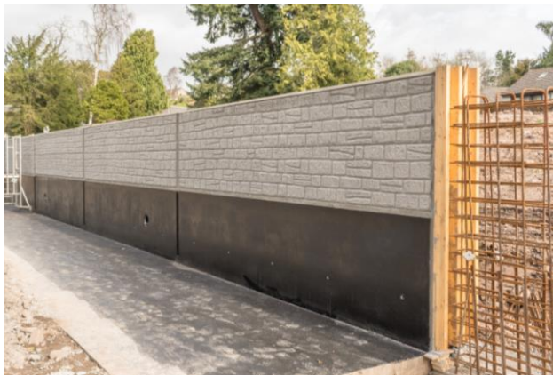
Trout Farm – Completion of reinforced concrete flood wall with aesthetic stone finish (black area will be below ground)
