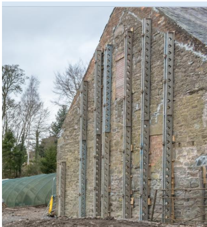
Trout Farm – Bracing of building
