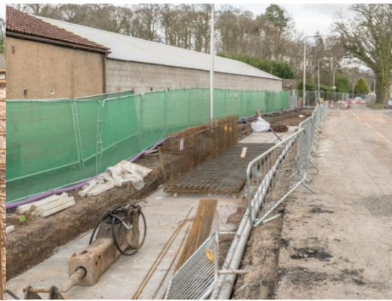
Lochty Park – Erection of reinforcement for retaining wall base
