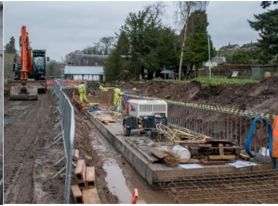
Trout Farm – Flood Wall concrete base complete and reinforcement erected for subsequent bases
