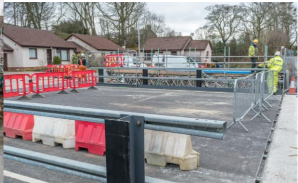
Lochty Park – installation of temporary bridge to allow demolition and construction of new Lochty Park bridge
