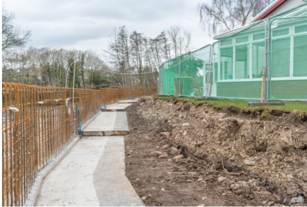
Druid's House – completion of flood wall bases and erection of reinforcement for flood wall stems.
