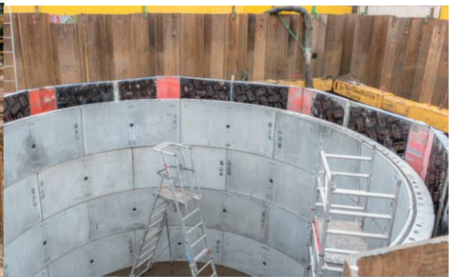
Vector – construction of pumping station chamber with concrete segments
