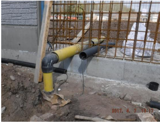
Druid's House – Not all services can be relocated away from the new flood wall. Some have to be designed into it.
