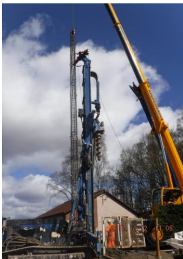
Lochty Park – construction of bridge piles. Lowering of steel reinforcement cage into the pile.
