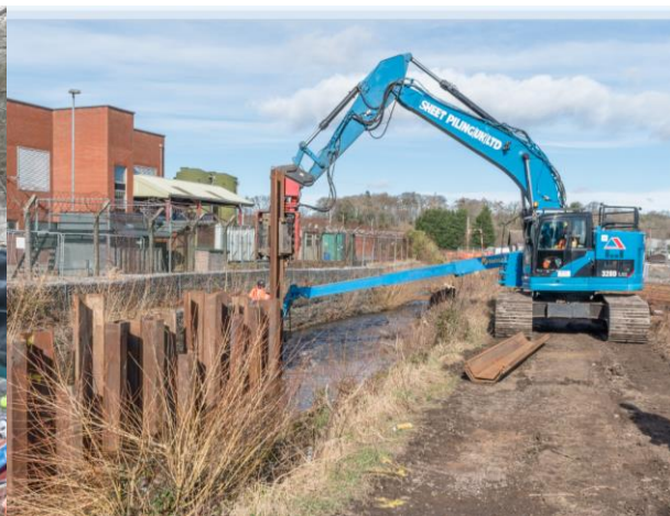
Puddledub – installation of temporary sheet piles in East Pow Burn for safe working and environmental reasons
