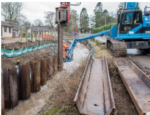
Lochty Park – Installation of temporary sheet piles for safe working and environmental reasons
