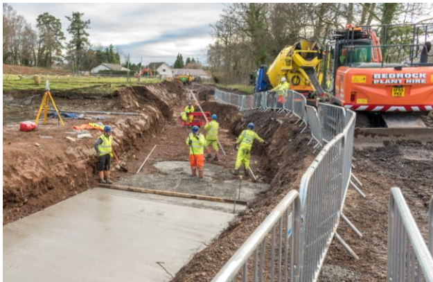
Trout Farm - Construction of blinding for flood wall base
