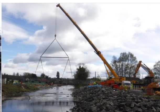
Black Bridge – relocation of black bridge in order to construct new bridge foundations
