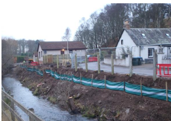
Lochty Park – Earthworks and erection of silt curtain to prevent discharge into burn
