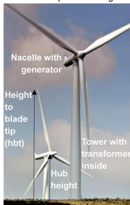
Figure 4.1: Wind turbine components © PKC
