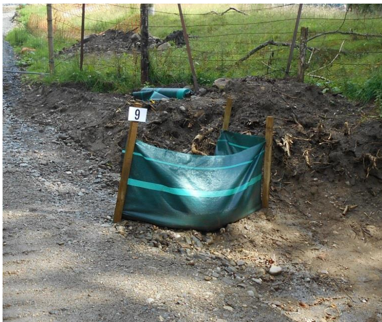
Effective silt trap, dug in, clearly numbered for maintenance ©PKC
