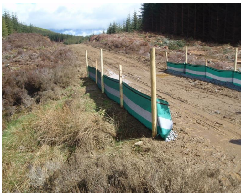
Splash guards at low points over river crossings or culverts ©PKC
