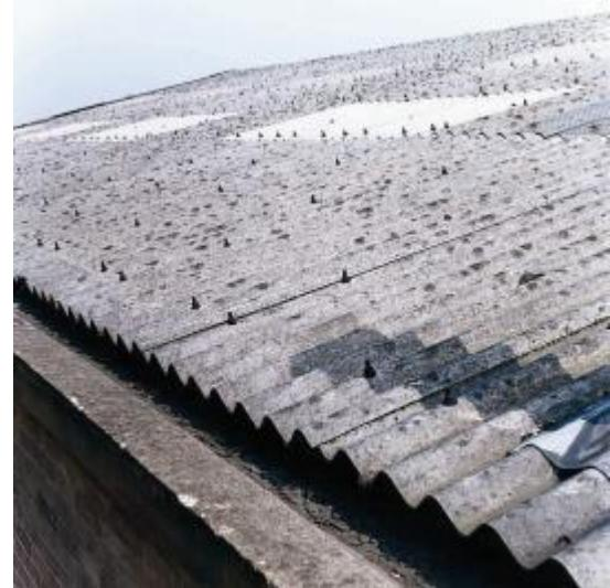
It was widely used in building materials from 1930 until about 1980, mainly to insulate properties and protect them against fire. Asbestos concrete was also used to make roof slates, rain water gutters, downpipes and decorative plaster finishes. This means that houses and flats built or refurbished in this period may contain some asbestos materials.
