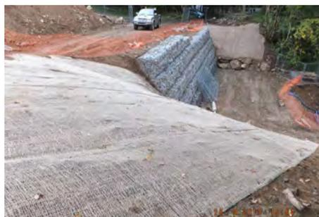
*Gabions and matting to protect soil during powerhouse construction*
