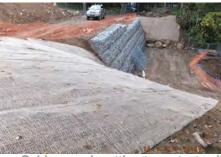
Gabions and matting to protect soil during powerhouse construction
