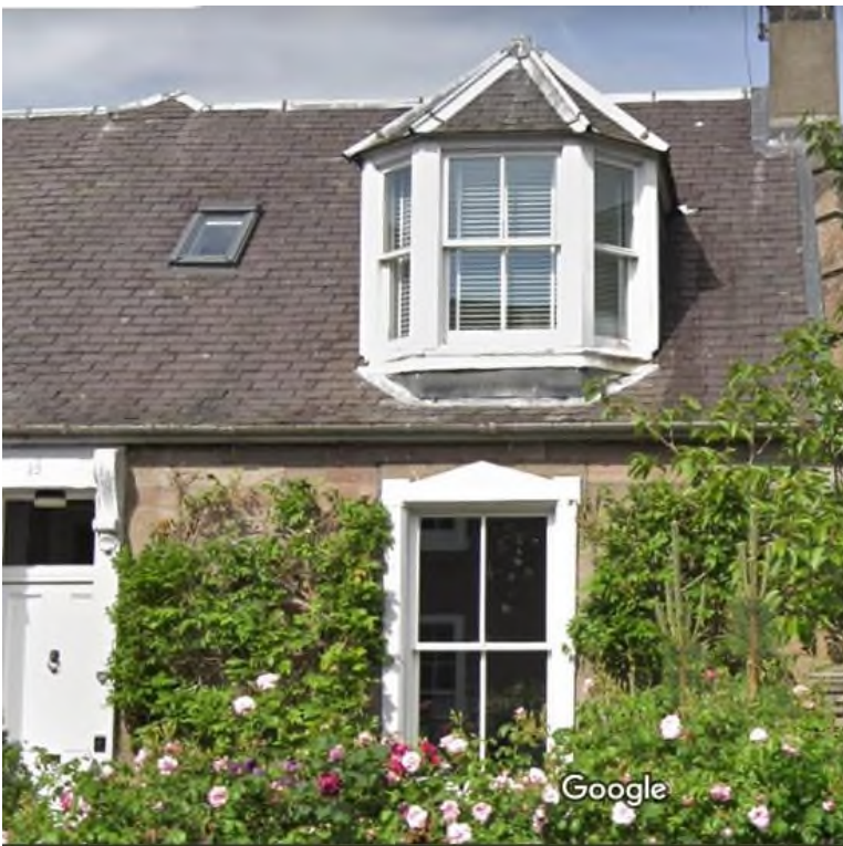
Single pane sash & case vertical sliding timber windows with centre astragal
