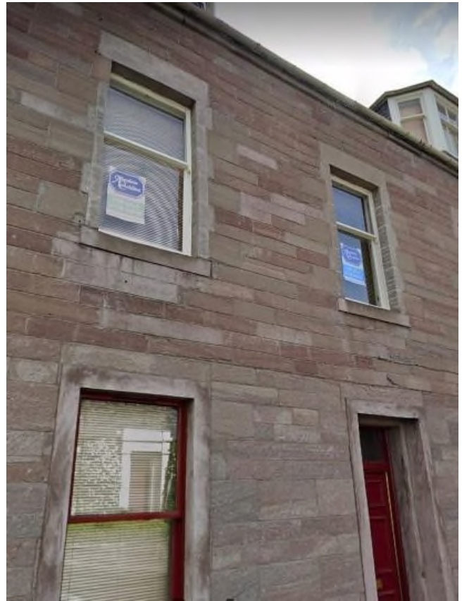
Timber sash & Case vertical slider – with no astragals no horns to ground floor and horns to first floor
