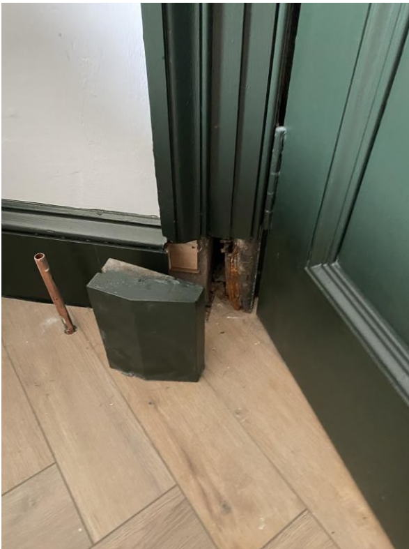
SECTION OF SKIRTING BLOCK REMOVED TO PROVE TO PLANNING DEPT WHAT ARE ORIGINAL SKIRTINGS.
