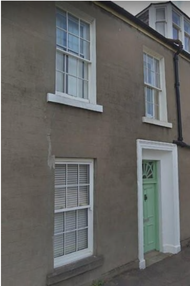
Timber sash & Case vertical slider – with plant-on astragals to ground floor and structural astragals to first floor
