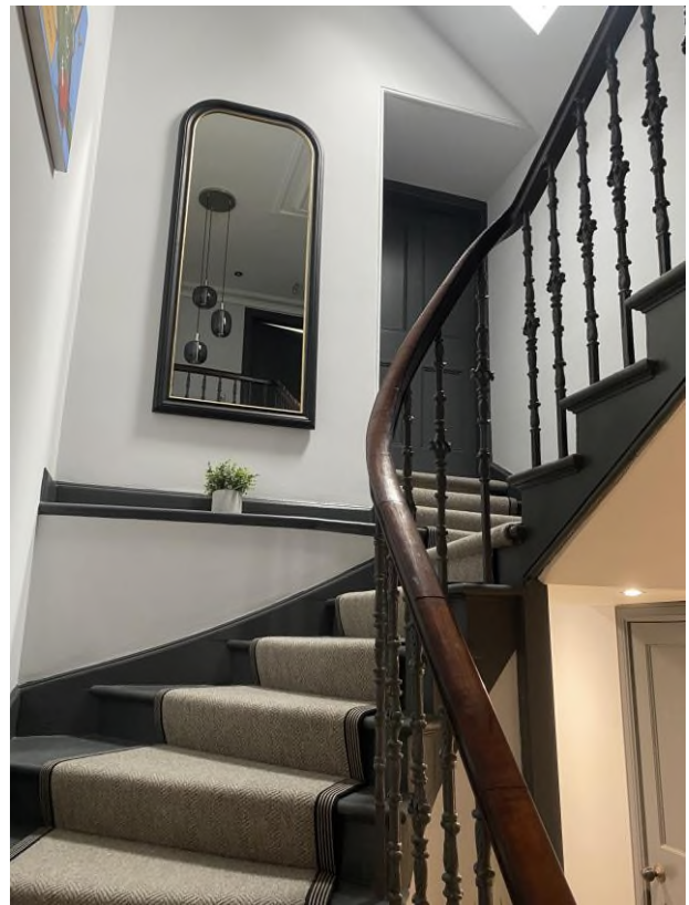
HALLWAY AND STAIRS RETAINED AND REFURBISHED WITH ALL ORIGINAL HANRAILS, BALUSTRADES, ARCHITRAVES AND DOORS RETAINED AND RESTORED
