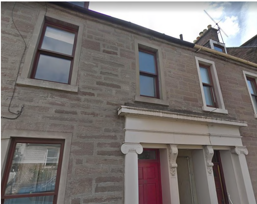
Timber sash & Case vertical slider – with no astragals
