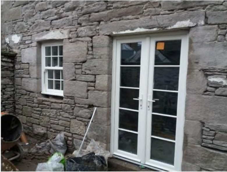
New Fitted W3 & D2 – White UPVC Framed Glazed Sliding Sash Window & White UPVC Framed Patio Door with Astragals.
