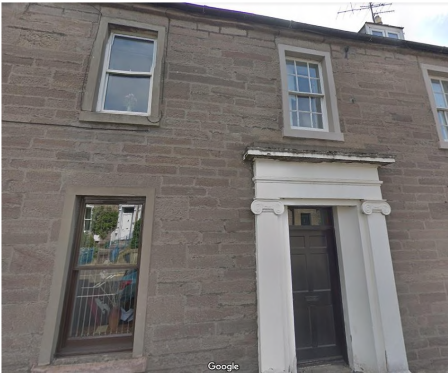
Timber sash & Case vertical slider – with no astragals and some 6 over 6 astragals
