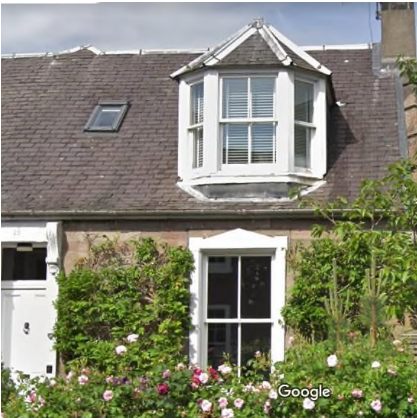
Single pane sash & case vertical sliding timber windows with horns
