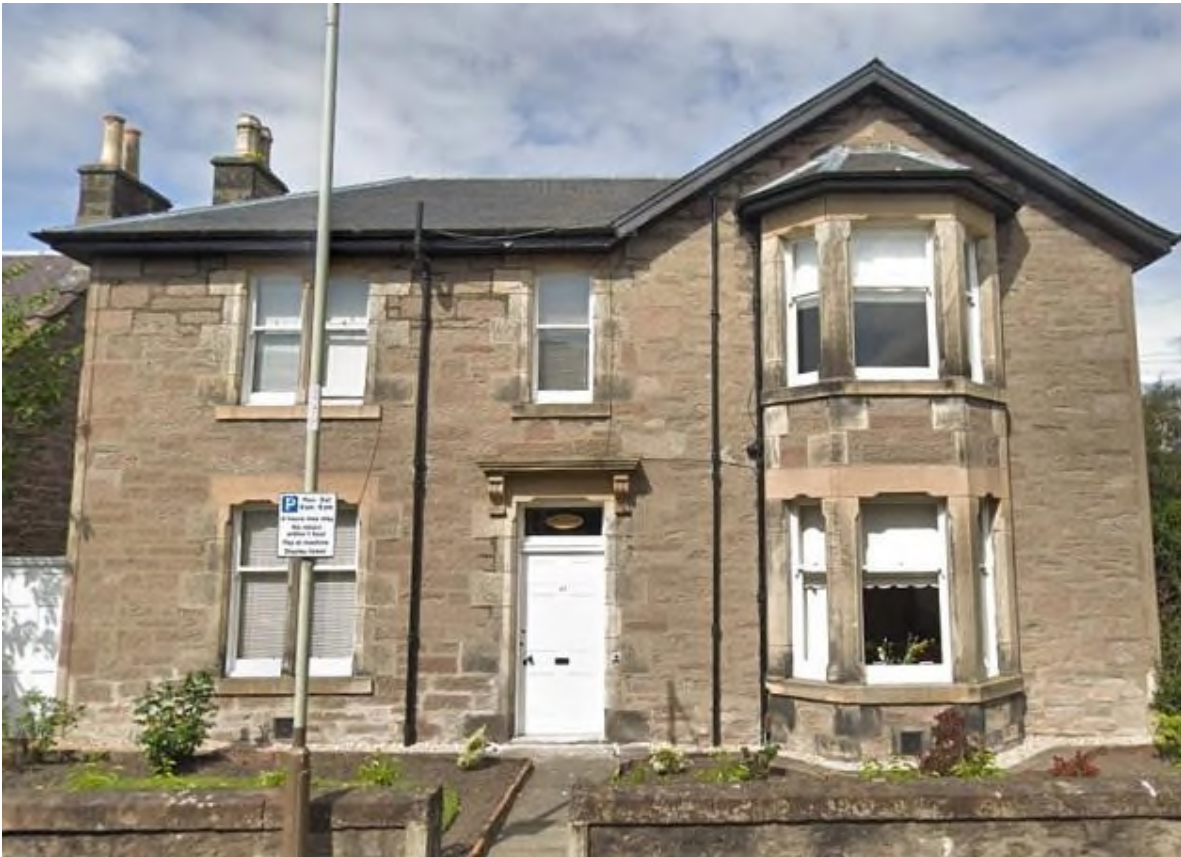
Single pane sash & case vertical sliding timber windows
