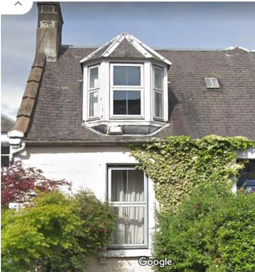
Aluminium mock S & C windows, casement opening
