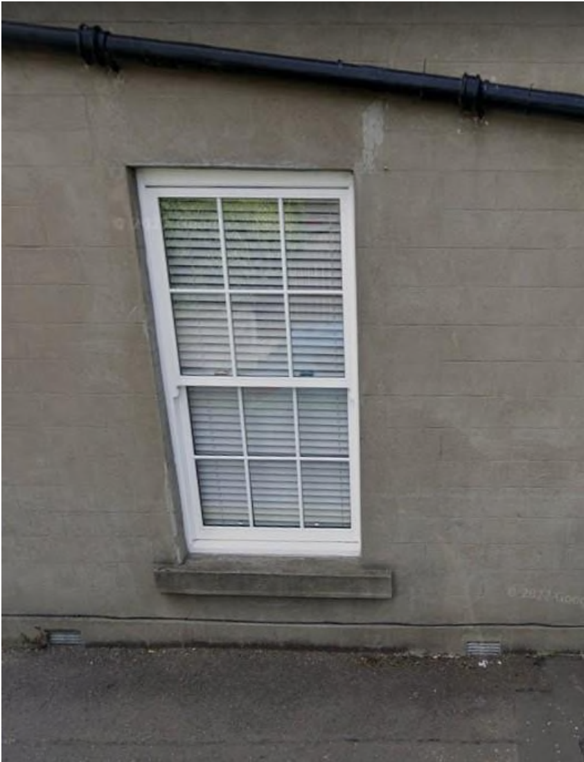
Timber sash & Case vertical slider – 6 over 6 with plant-on astragals
