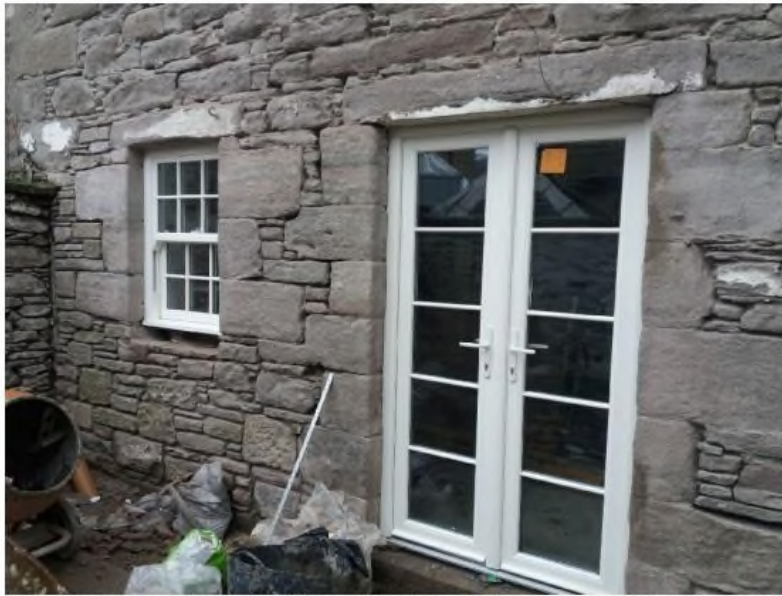
New Fitted W3 & D2 – White UPVC Framed Glazed Sliding Sash Window & White UPVC Framed Patio Door with Astragals.
