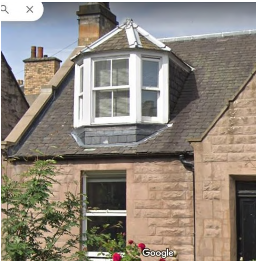
Timber sash & Case vertical slider – with plant-on astragals
