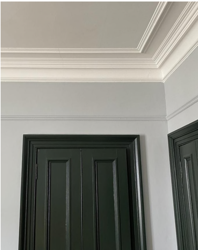
LOUNGE AFTER STRUCTURAL REPAIRS AND CORNICE RESTORED AND ROOM REPAINTED
