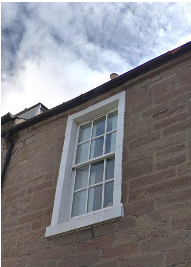
uPVC sash & Case vertical slider – 6 over 6 with plant-on astragals
