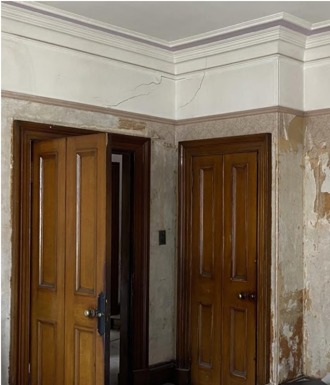
ORIGINAL LOUNGE WITH STRUCTURAL CRACK THROUGH WALL AND CORNICING
