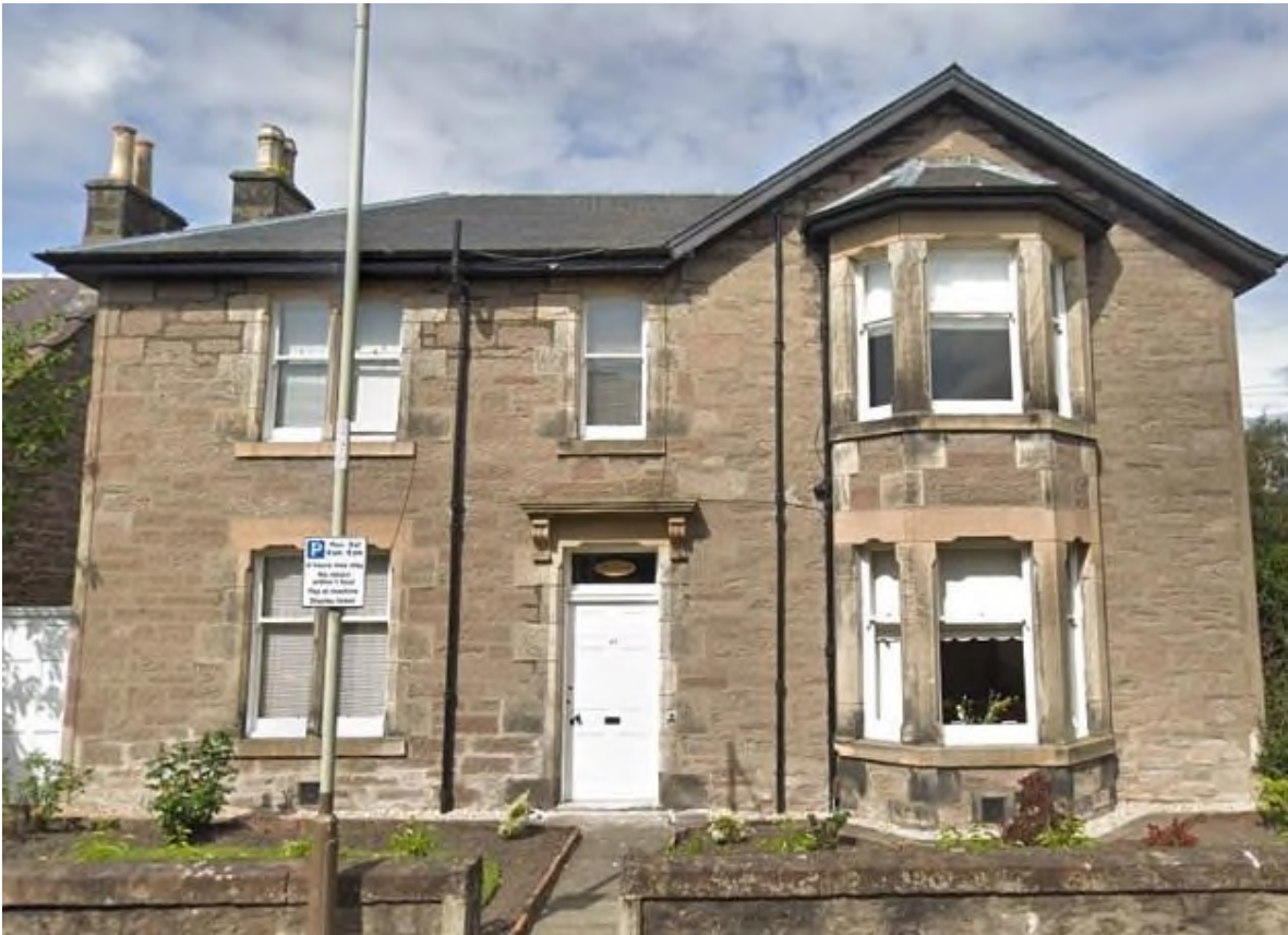
Single pane sash & case vertical sliding timber windows with horns
