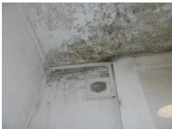
Damp and mould to the bathroom ceiling.
