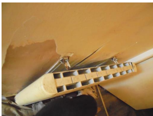
LHS hall radiator bracket has failed.
