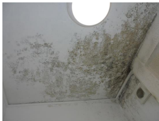
Damp and mould to the bathroom ceiling
