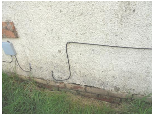
The foundation blockwork read as being damp, moss evident and some bossed harling. Cavity fill holes.
