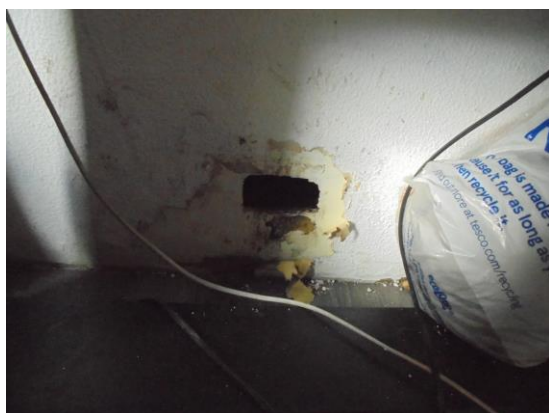
Missing vent cover to chimney vent in living room.
