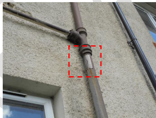
Front waste water pipe, hole repaired with flashing.
