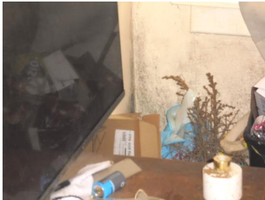
Bedroom 1 inside of the exterior wall, area read as being damp
