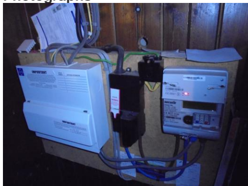
Electric consumer unit and meter.
