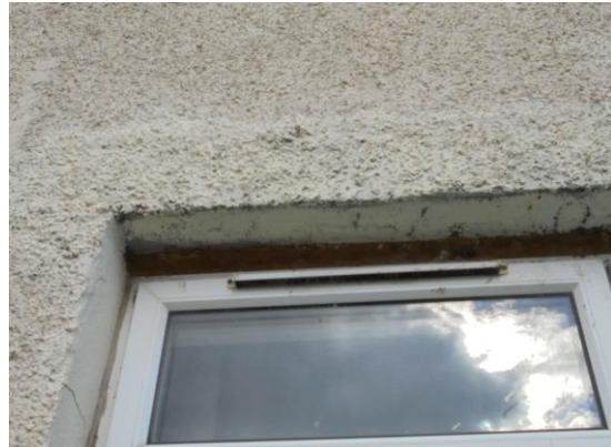
Exposed expanding foam between top of window frame and new lintel.
