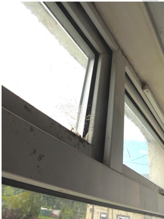
Opening fan windows, not shutting to stops.
