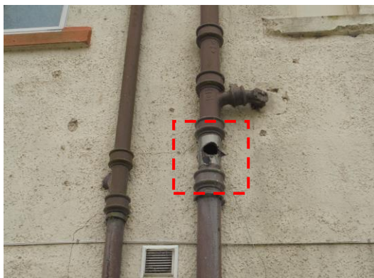
Hole exposed in waste water pipe, gable.
