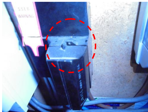
Missing main fuse security tag.
