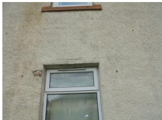
Back bedroom 1 lintel, showing signs of cracking at the lintel area.
