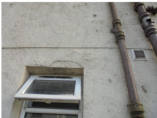
Gable bathroom lintel, showing bossing of harling at lintel area.
