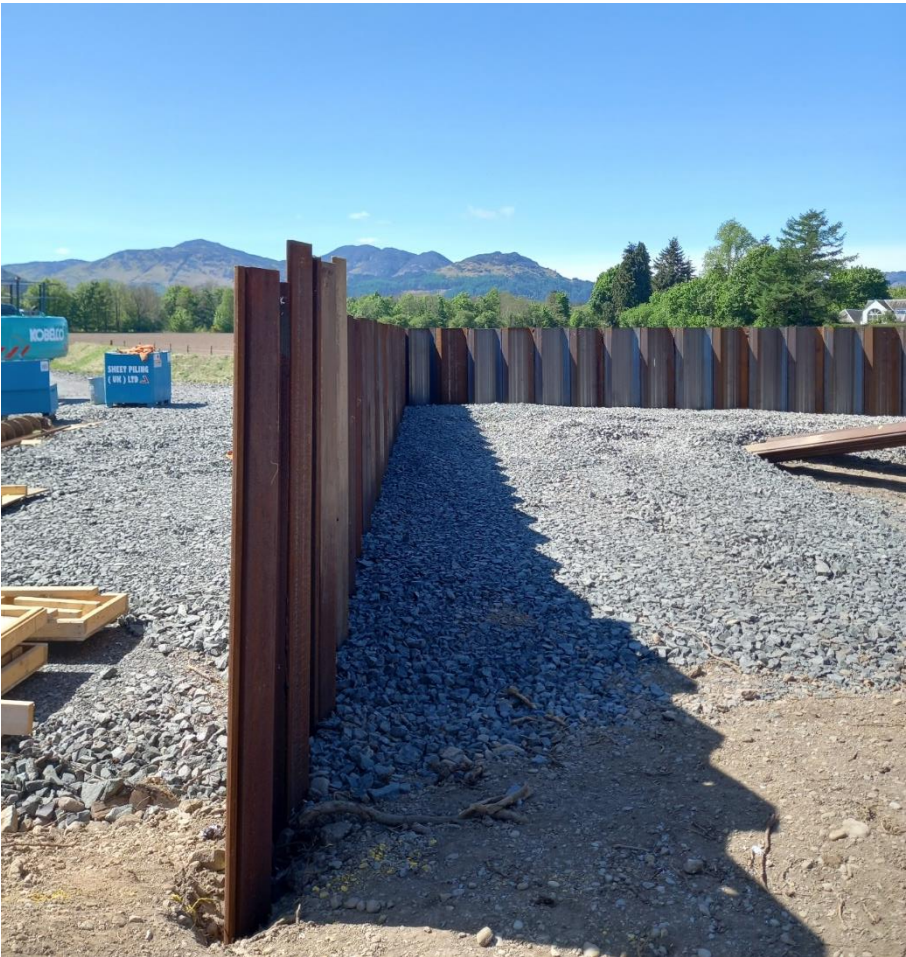
Steel sheet piles at Aros field looking west - these form the core of the new flood embankment (6 May 2025)
