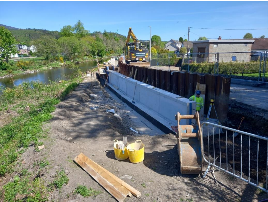
Formation of first section of reinforced concrete flood wall at Strowan Road, with seepage cut off piles to the rear (to be cut down below road level) (6 May 2025)
