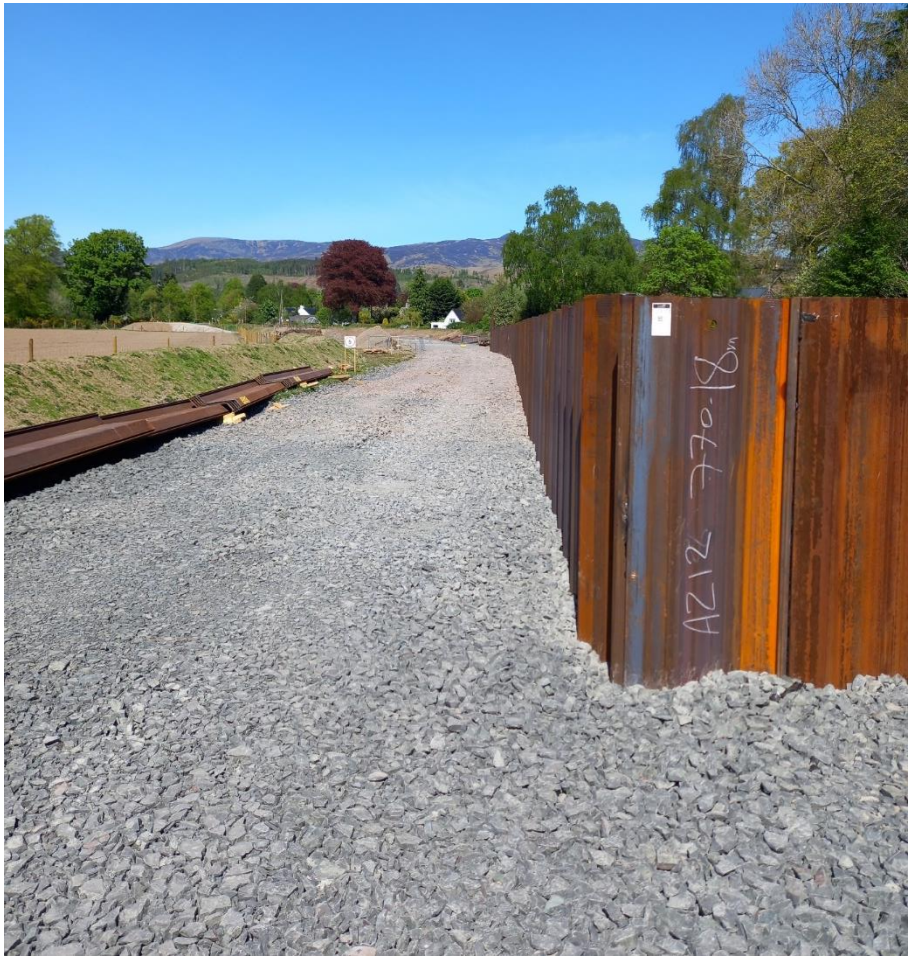
Steel sheet piles at Aros field looking north to Camp Road - these form the core of the new flood embankment (6 May 2025)
