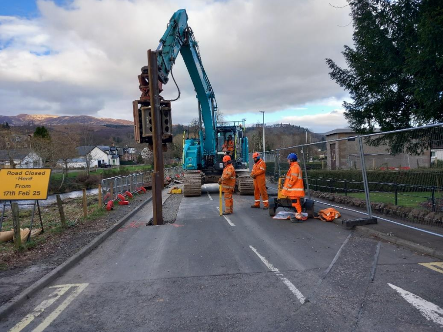
First sheet pile installed at Strowan Road - these piles will provide a below ground seepage barrier and be cut down below road level (10 March 2025)
