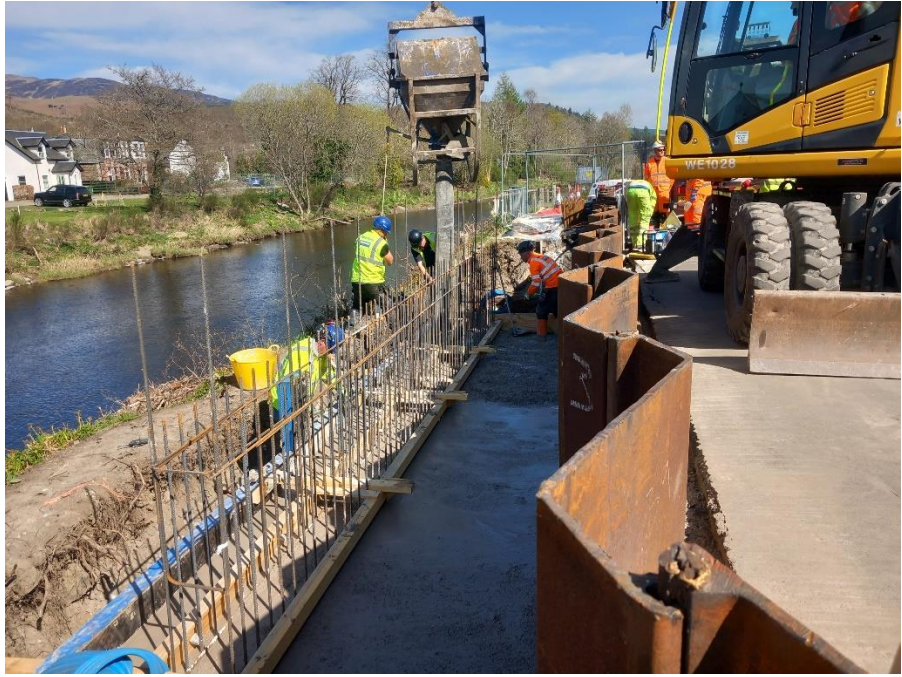
Concrete pour for reinforced flood wall at Strowan Road (11 April 2025)
