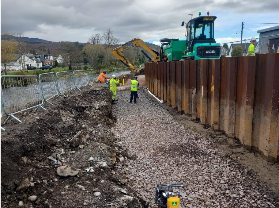
Formation of base level for flood wall at Strowan Road (31 March 2025)
