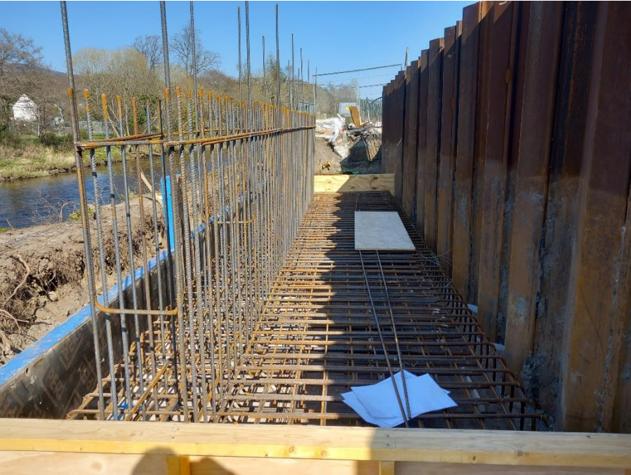
Preparation of wall reinforcement prior to concrete pouring at Strowan Road (8 April 2025)
