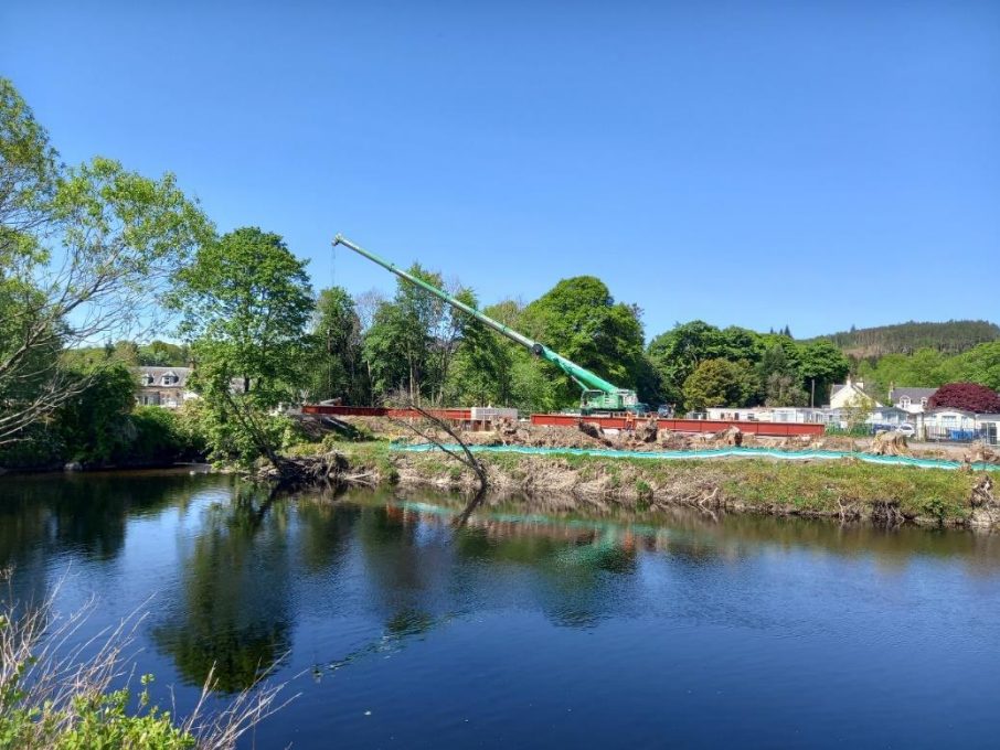
Installation of temporary construction vehicle bridge over R. Lednock (6 May 2025)
