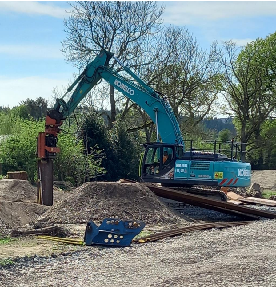
Installation of first steel sheet-pile at Aros Field (30 April 2025)
