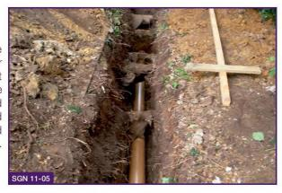
Ducting services that have to be threaded through existing roots is good practice because it reduces the need to excavate in the future. Note the hessian protection over roots while they are temporarily exposed to prevent sunscorch and drying.
