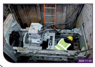
Thrust boring is the preferred option for installing service routes through the RPAs of retained trees.
