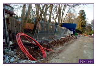
Conventional installation of services digging a trench with a machine is **not permitted** in RPAS.
