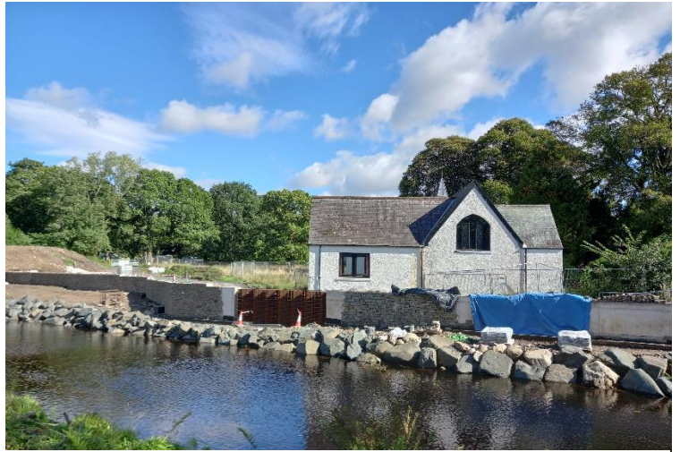
Flood wall at St Serf's Church under various stages of construction (16 September 2025)
