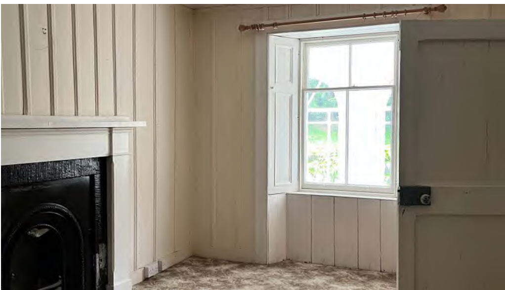
Former West Cottage - Proposed Home Office / Study Existing timber panelling to be repaired as necessary and re-painted
