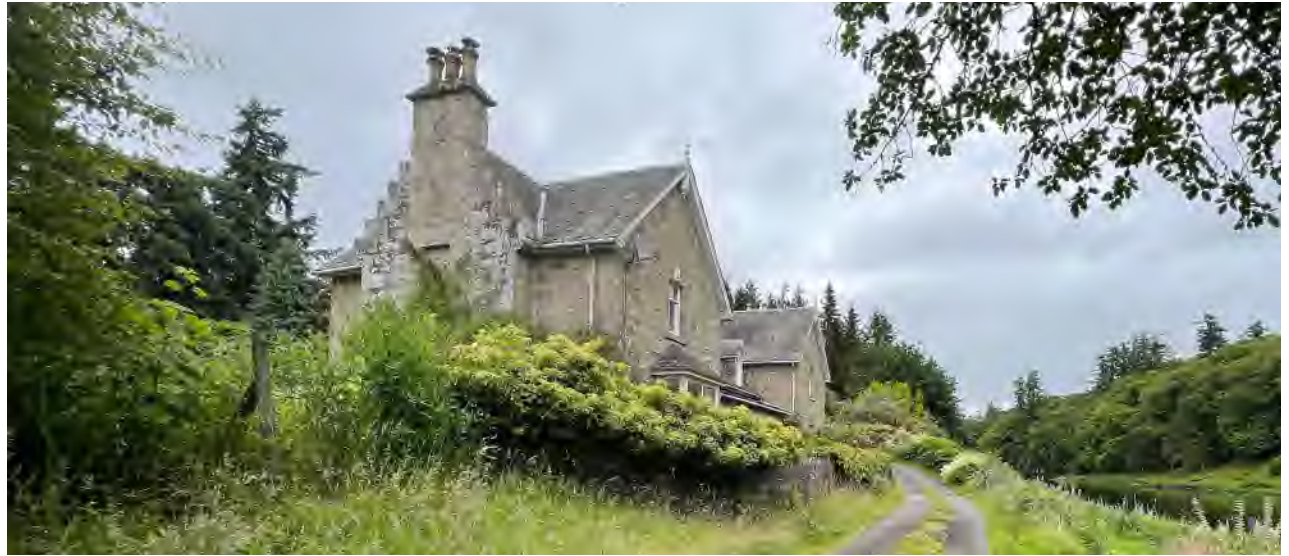
View on approach, as existing - Photograph [July '24]
