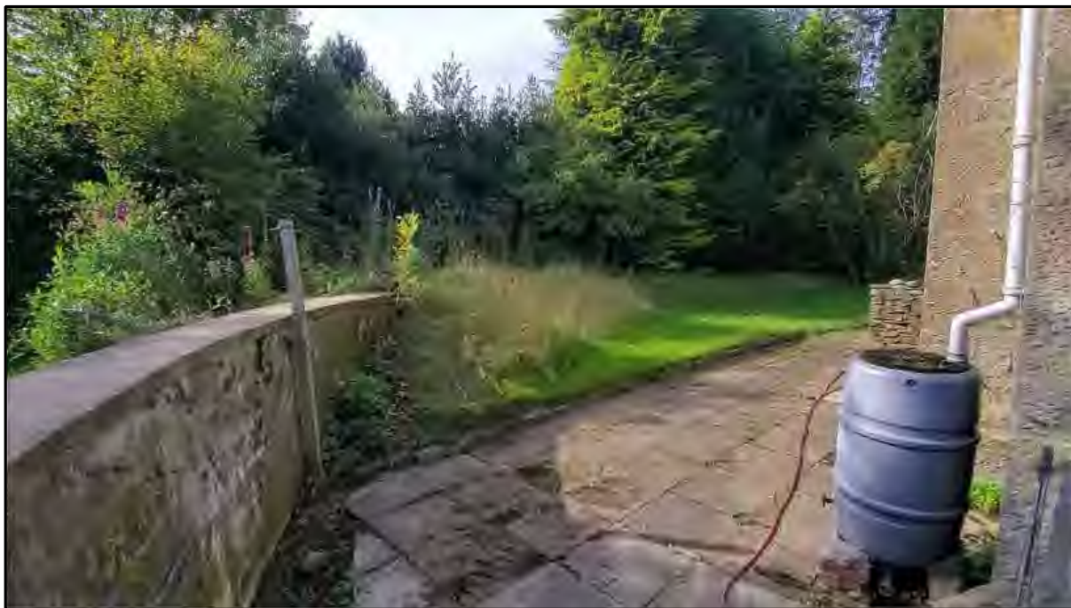
Photograph 7 - Looking northwest along the flood wall and the connecting flood bund behind, from the southwestern corner of the house.
