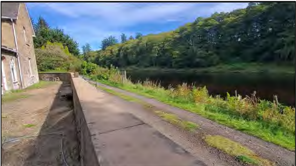
Photograph 6 - Looking east (downstream) along the flood wall, with the main frontage of the house on the left, and access track and the River Tay to the right.
