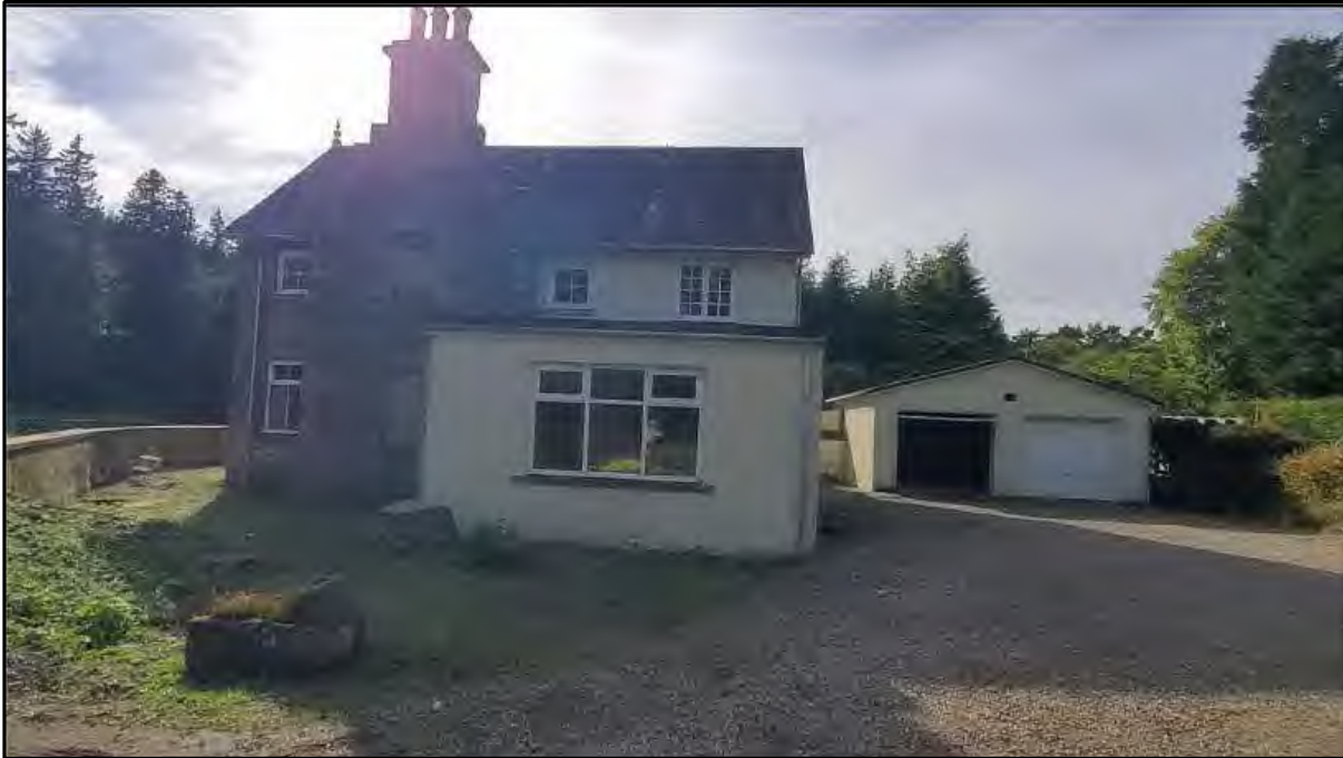
Photograph 1 - Boat of Murthly main house in centre, annexe building to the right/behind, and flood wall to the left. The annexe building on this side is a double garage, whereas the western side of the annexe (see Photographs 9 and 10) is a wooden clad building which includes a toilet and a shower room.
