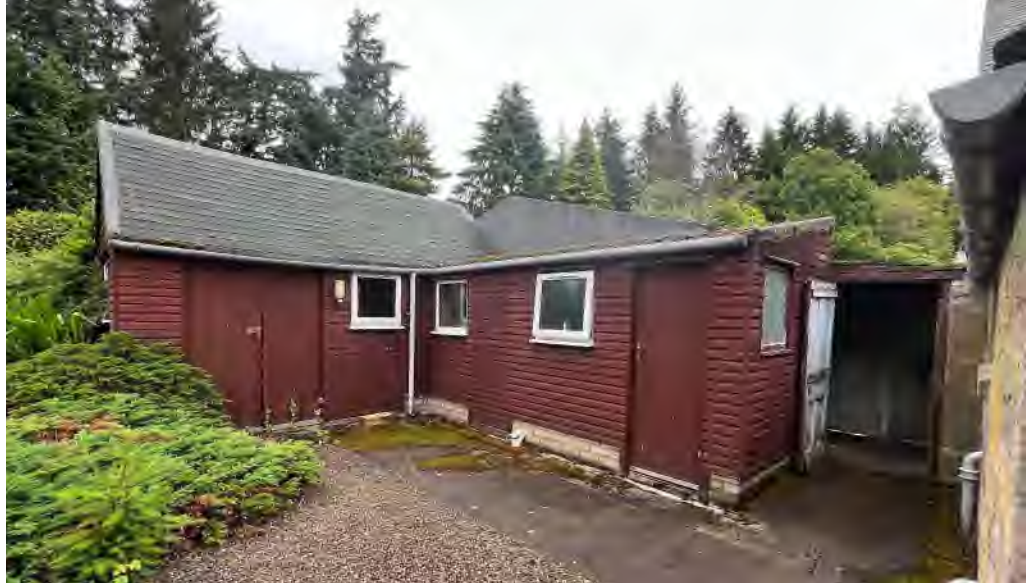
Existing rear accommodation including workshop space
