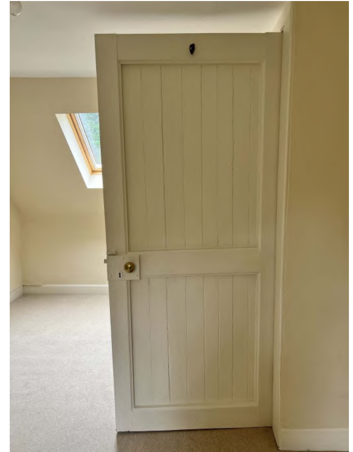
Existing Internal Doors to be retained.
