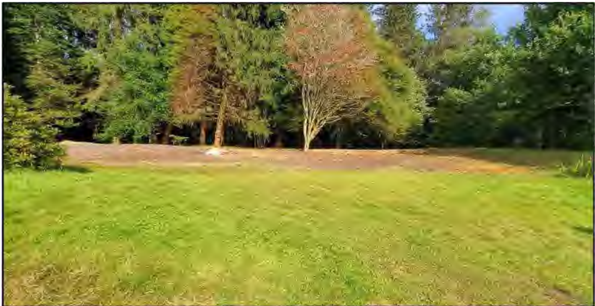
Photograph 11 - Looking east to higher ground. On the right, the downstream flood bund which connects between the flood wall and higher ground can be seen tapering to zero (area in shadow on right below trees).
