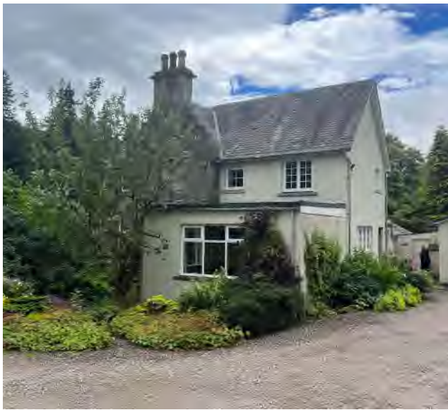
Existing 1970's extension
