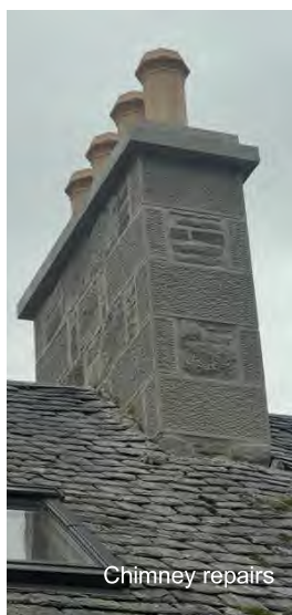
Recent repointing work
