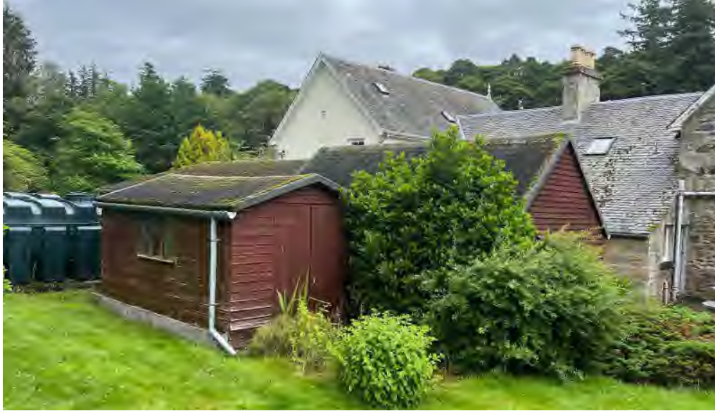
Existing rear accommodation
