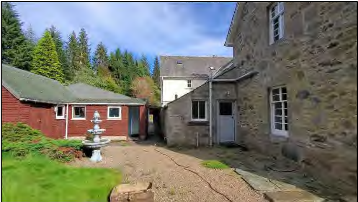
Photograph 9 - Rear of the main building on the right, and annexe building on the left.
