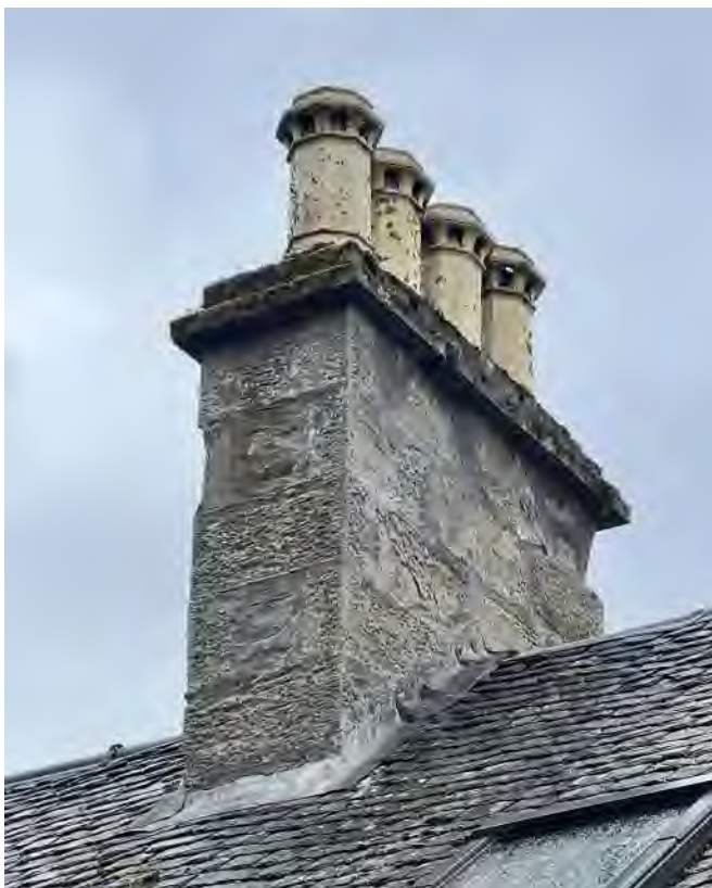
1no. of 3no. existing chimneys to be taken down and rebuilt as part of separate listed building consent application.
