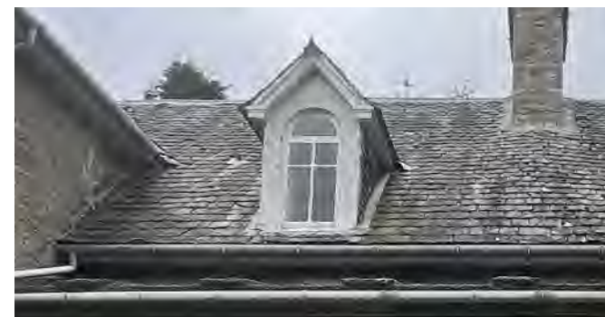
Window Type 3 - Existing Dormer Windows
