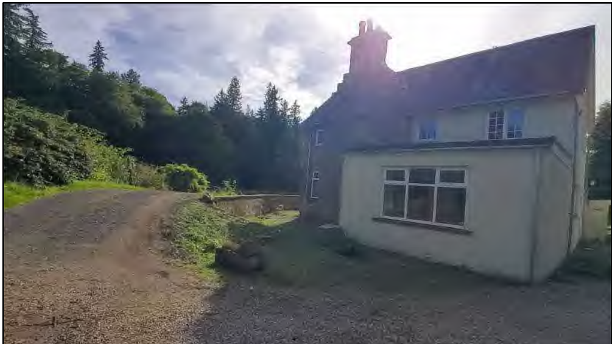
Photograph 2 - Main part of house in masonry with existing extensions (yellow render) to the right. Access track on the left as it drops down from high point over flood wall.
