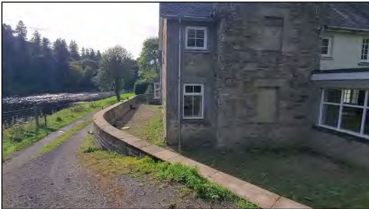
Photograph 3 - Main part of the house, with existing extensions to the right, and flood wall/river to the left, viewed from the high point on the access track.
