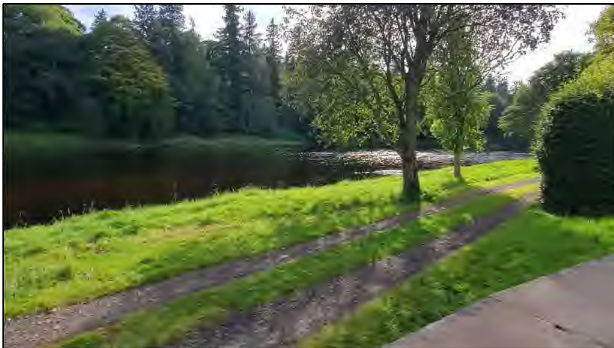
Photograph 8 - View from the upstream (western) end of the flood wall, towards the access track and the River Tay beyond.
