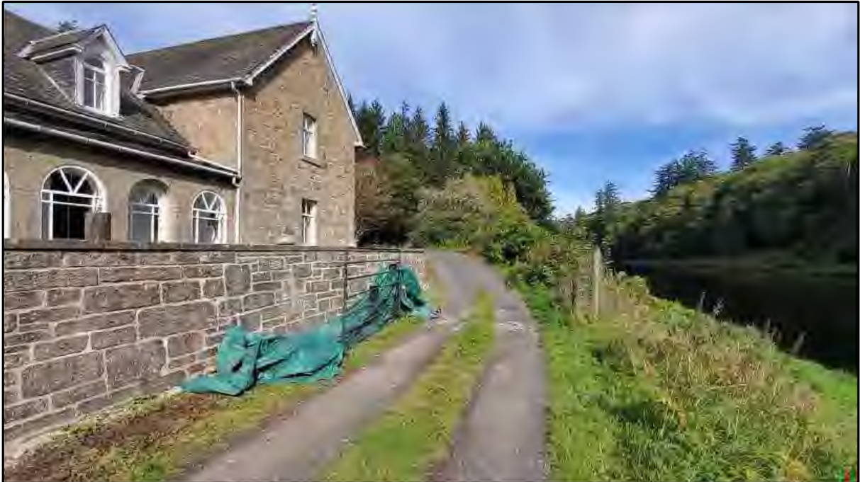
Photograph 5 - Eastern end of the house, with the access track rising up to cross over the top of the flood wall.
