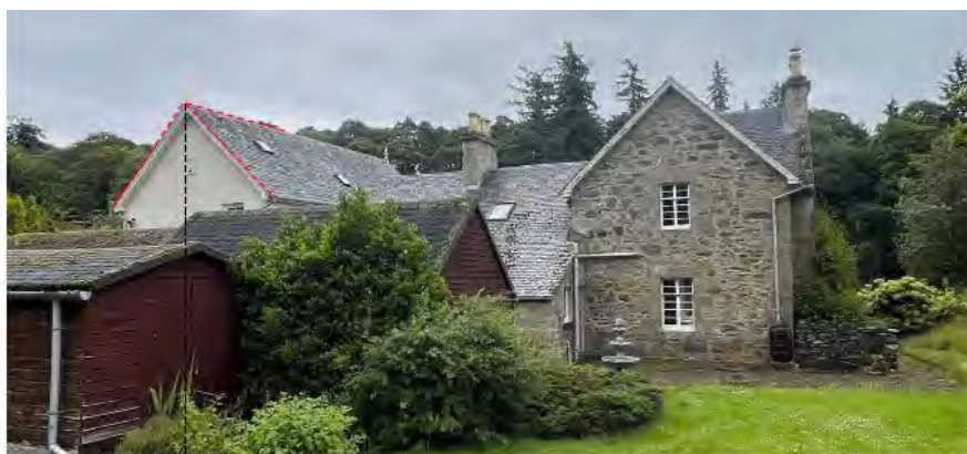
View from rear, as existing - Photograph [July '24]
