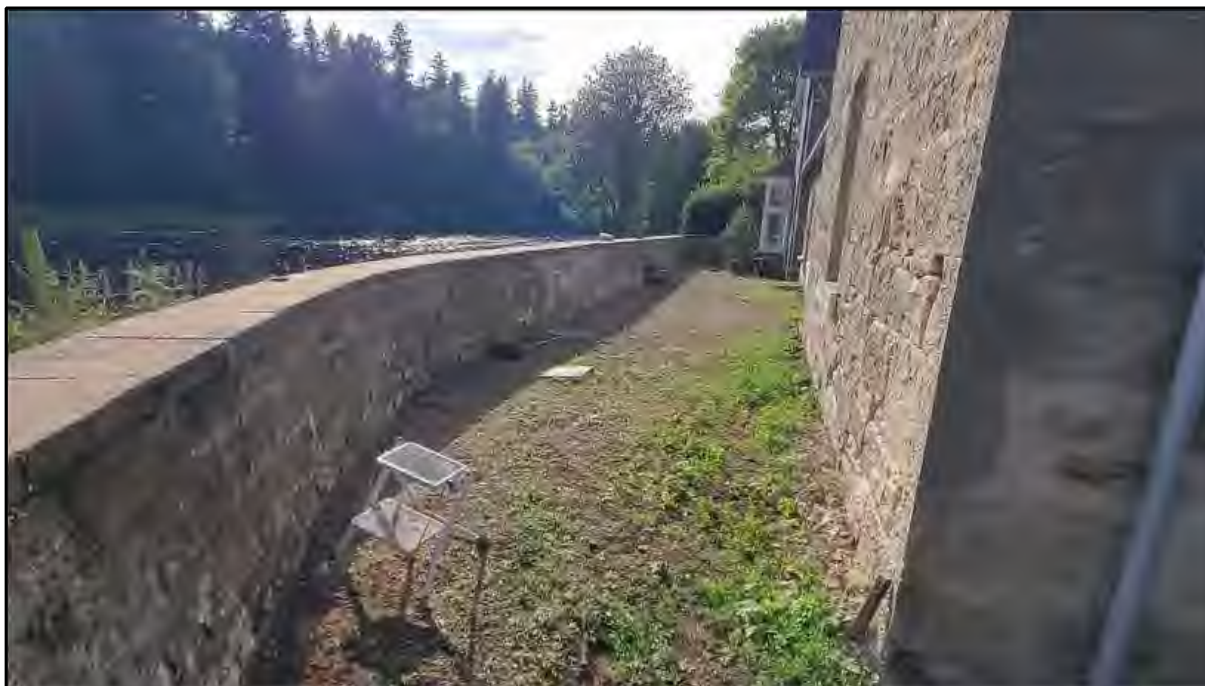
Photograph 4 - Looking west (upstream) along the flood wall and the River Tay beyond, from the southeast corner of the house.
