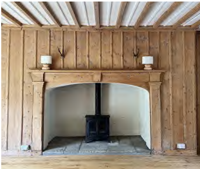
Large inglenook fireplace in principal rooms to be retain
