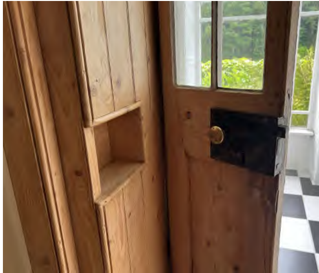
Existing Former External Doors to South to be retained
