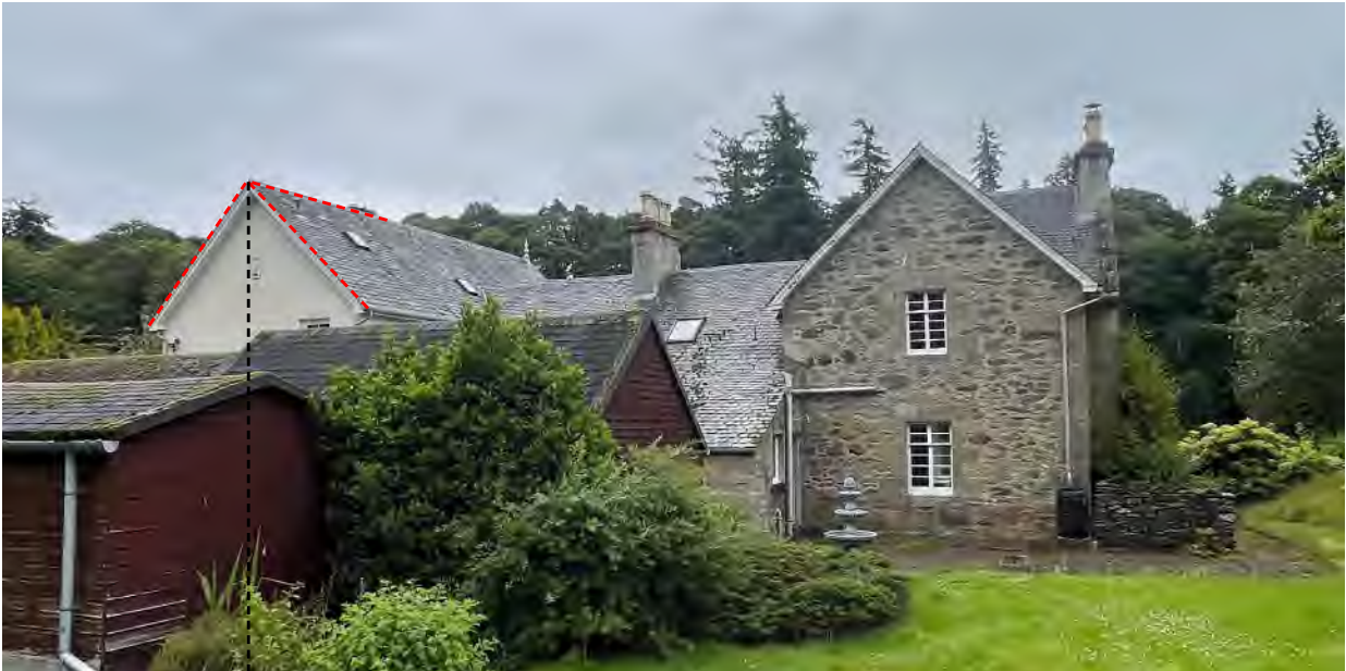
View from rear, as existing - Photograph [July '24]
