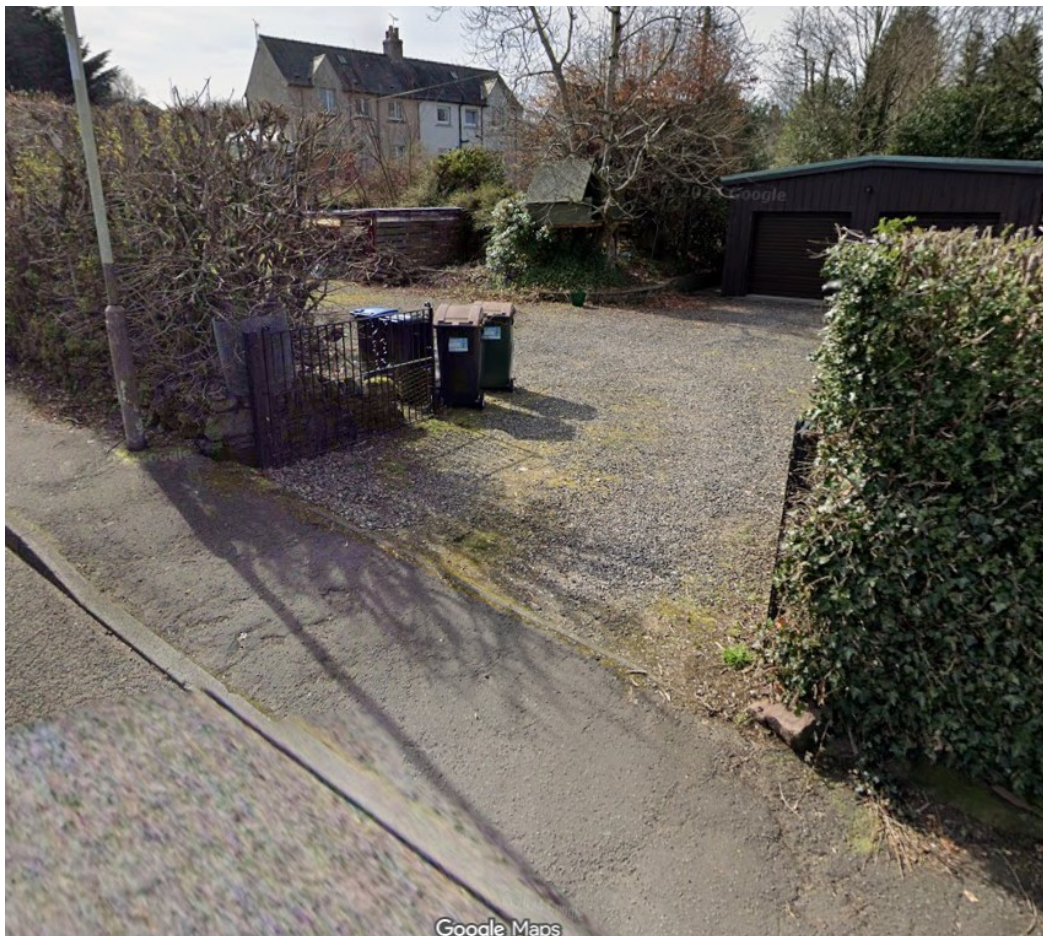
Access at Highfield, neighbouring property to north. Narrower than proposed access for 25/01754/FLL. No lowered hedge or pedestrian splay.
