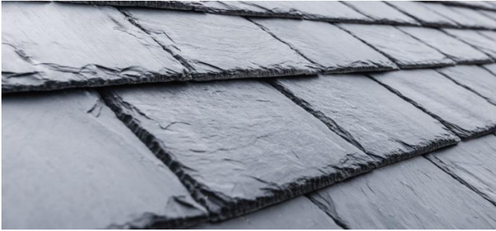
Natural Slate Roof
