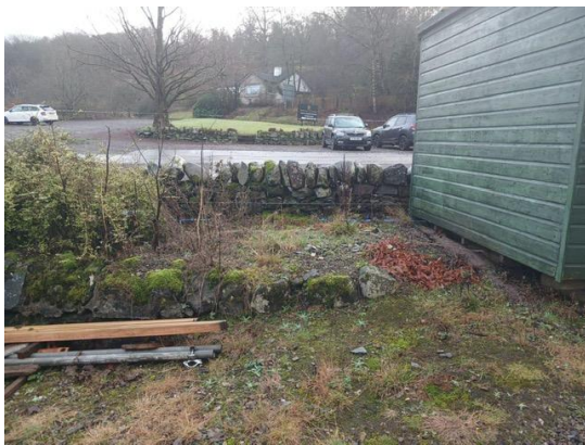
Extract 10 – Looking into carpark
