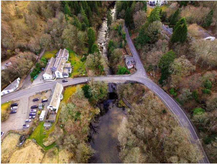
Extract 6 – Ariel view of bridge and application site
