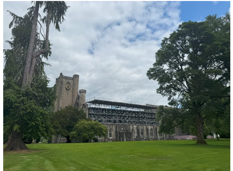
Figure 24 – Dunkeld Cathedral with scaffolding
